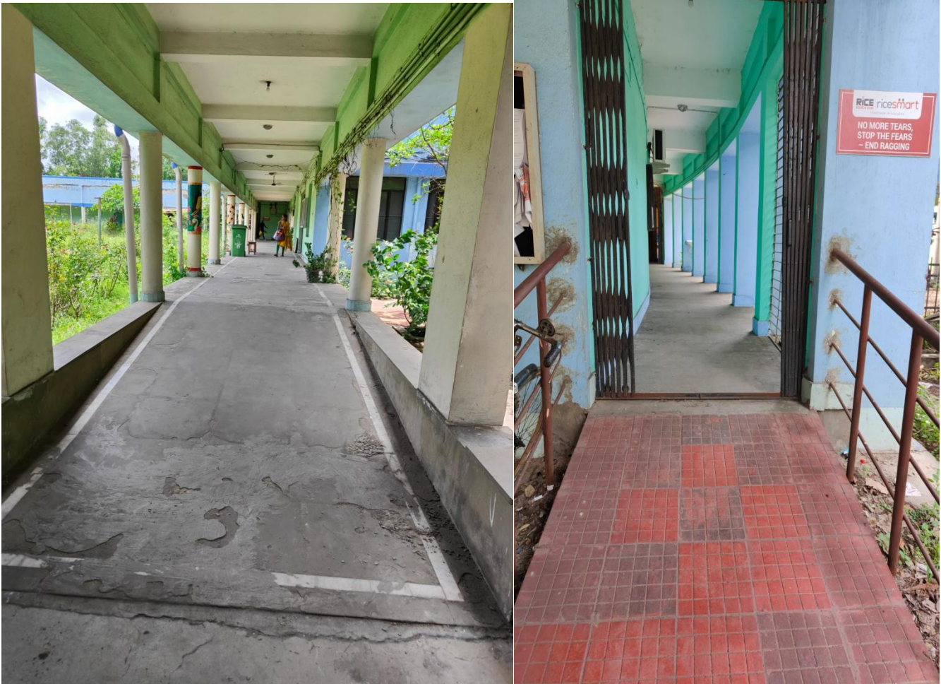
Disabled Friendly Ramp (Photograph taken on 11/06/2023)
